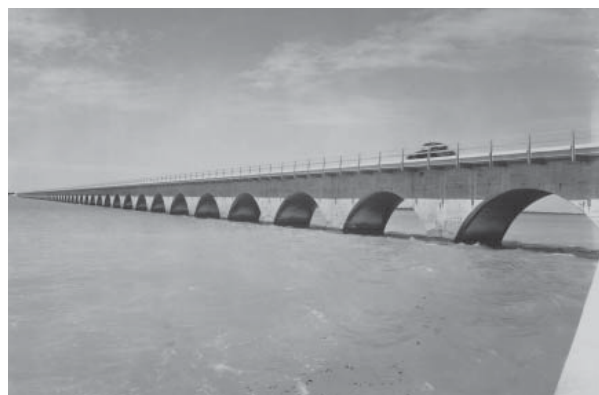
Fig. 3 View from ground showing the widened railroad bed for automotive traffic at Matecumbe Key. NARA, 1938.
