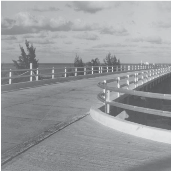
Fig. 4. Rails reused as guardrails on new portion of Overseas Highway to Key West. NARA, 1938.
